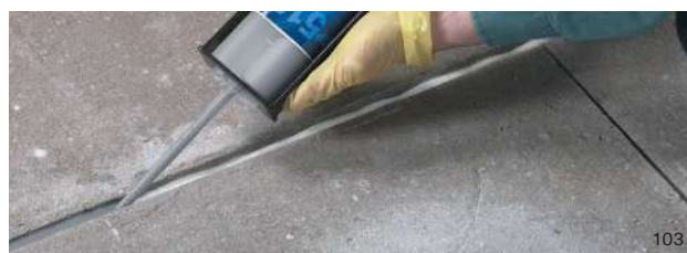
Make fast work of lengthy expansion or control joints and other larger jobs with the heavy-duty manual applicator and 12 fl oz. duo-pak cartridges.
